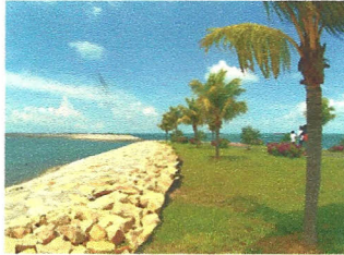
Southern side of the landfill
